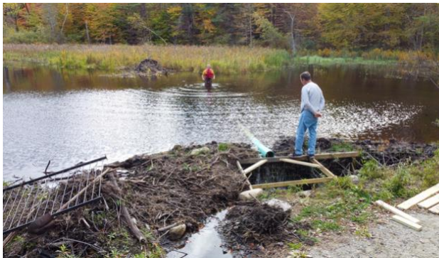
A Beaver Dam Near a Halifax Road Being Outfitted with a Beaver Deceiver © Skip Lisle (photo: David Erickson, Halifax VT)
