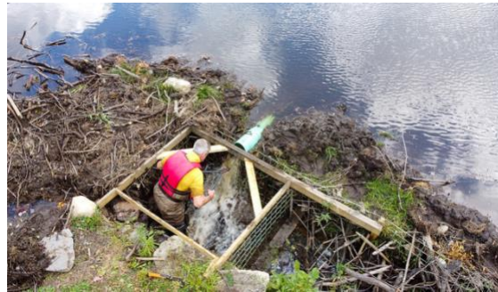
Installation of a Beaver Deceiver © Skip Lisle (photo: David Erickson, Halifax VT)
